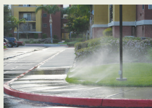
Runoff from overspray or excessive irrigation
