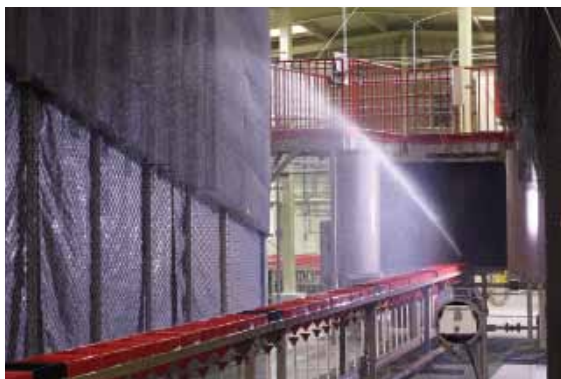
Extensive testing for T5 nozzle efficiency was performed using SPACE calculations
